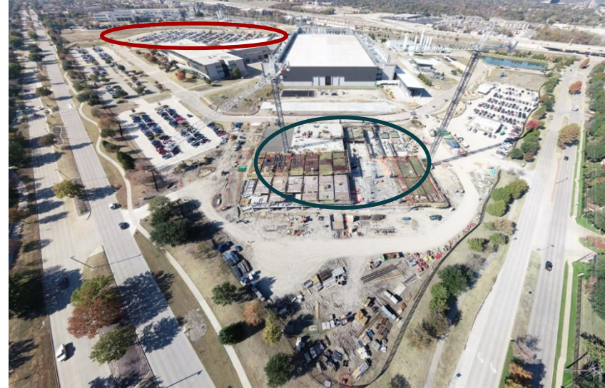
Existing factory and parking garage construction underway
